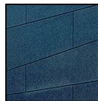
4 ALUMINIUM CLADDING: ALUCOBOND DARK GREY METALIC
