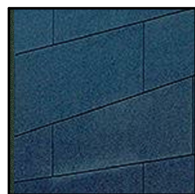
4 ALUMINIUM CLADDING: ALUCOBOND DARK GREY METALIC
